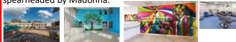
Far left: Exterior, nearly complete. Second from left: Atrium mural, "Tree of Life" by Jacaranda Home for Children. Second from right: Mandela mural by Kobra. Right: One of three operating 'theatres'.
